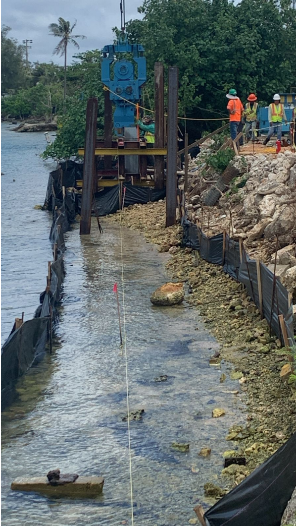
Coop Seawall Construction
